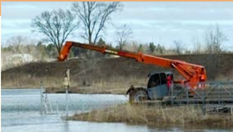
Permanent pier installation at Oneida Lake.
