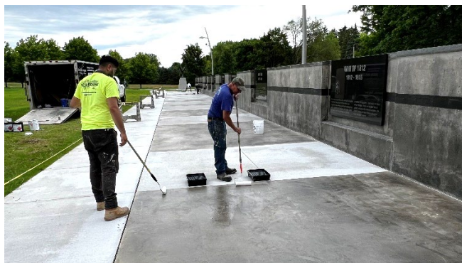
VETERANS MEMORIAL CONCRETE STAINING
