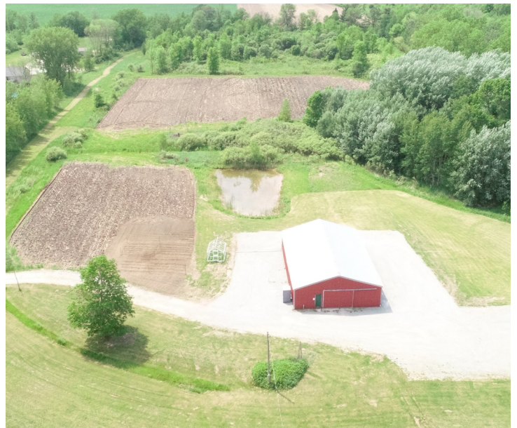
Picture 3: 4-H Project completed
