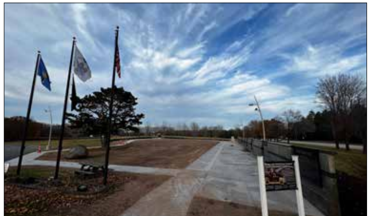
▲ Finished accessible concrete paths at the wall.
