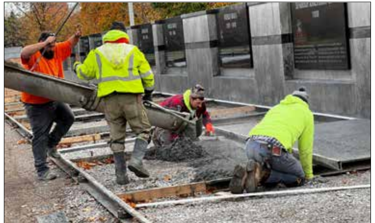
▲ Crew pouring concrete paths at the wall.
