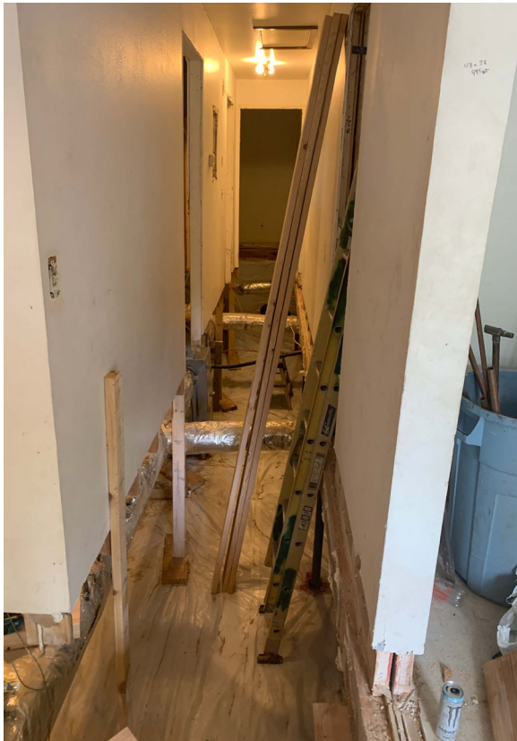
Home renovation: Hallway
