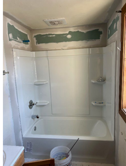
After Bathroom repairs
