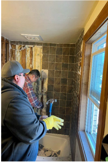
Before Bathroom Repairs
