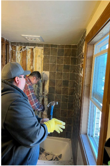
Before Bathroom Repairs
