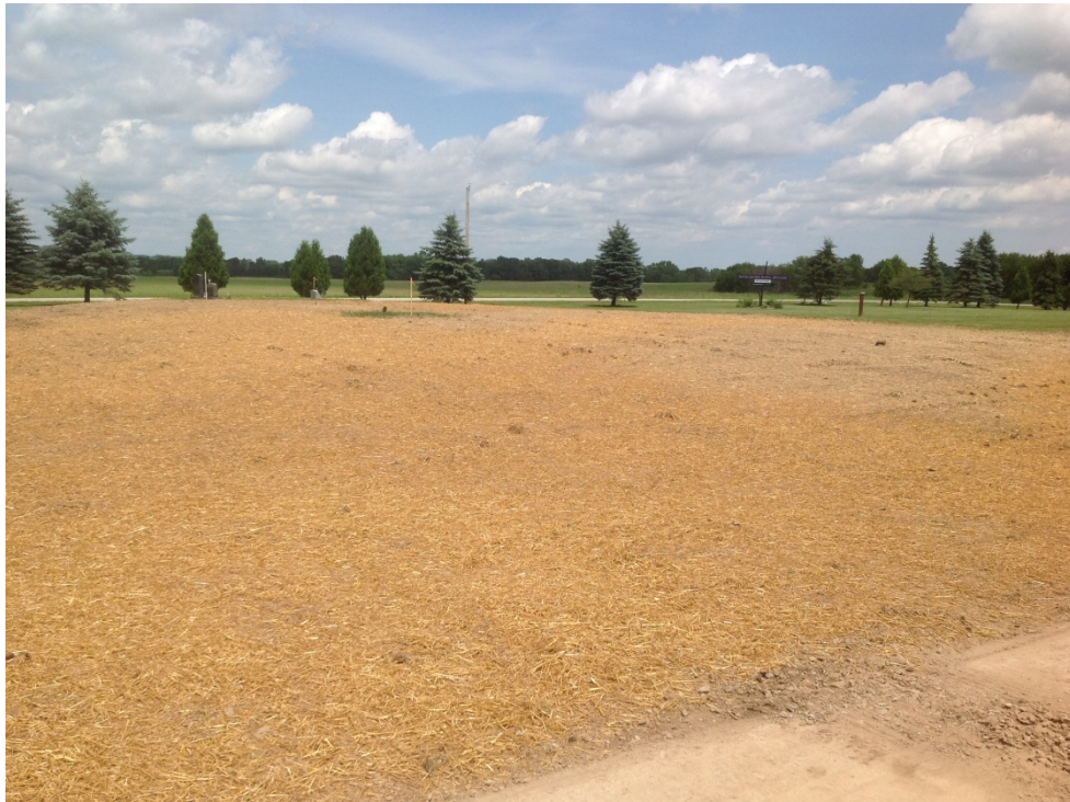
Sections D & E complete (looking northeast)
