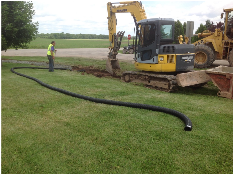
French Drain along west entry road being installed
