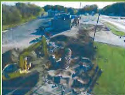
October The 54 One Stop underground storage tank removal and building demolition.
