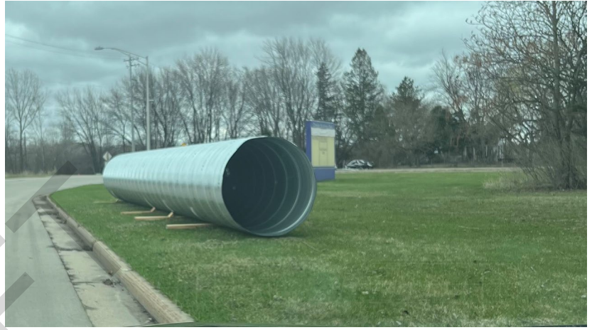
Replacement culvert for the Duck Creek Trail
