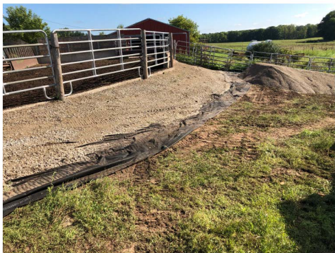
Improved Barnyard at Tsyunhehkwa to Reduce Runoff
