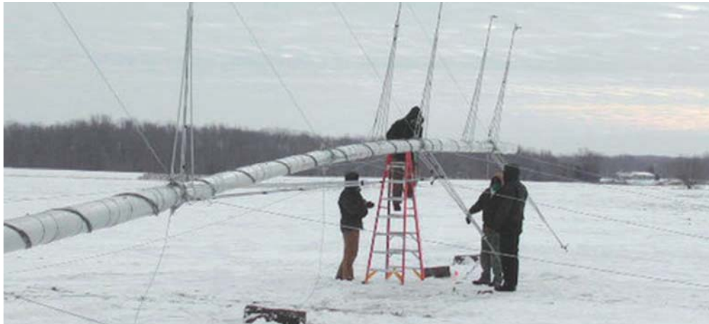
Installation of Wind Monitoring Tower in December 2009
