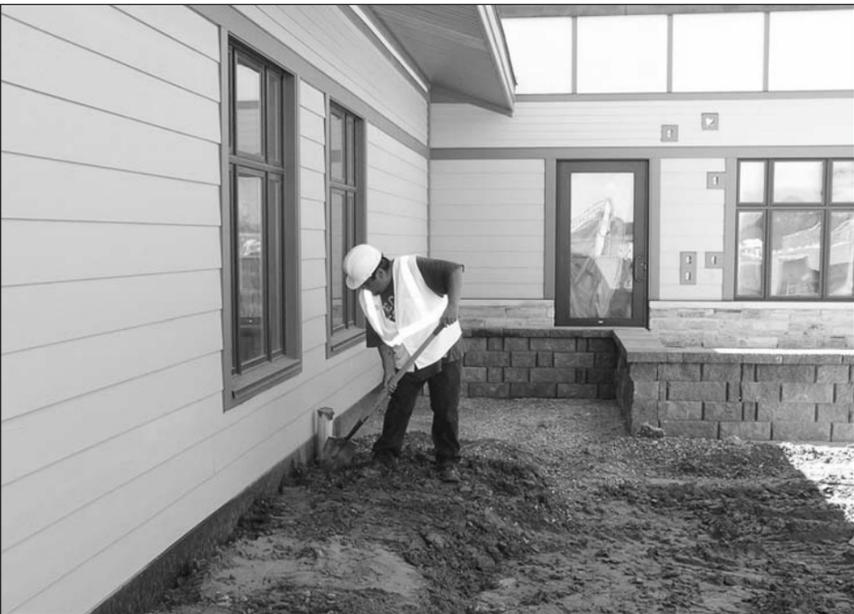
Hartman Skenandore of Gauthier Construction backfilling around a storm drain.
