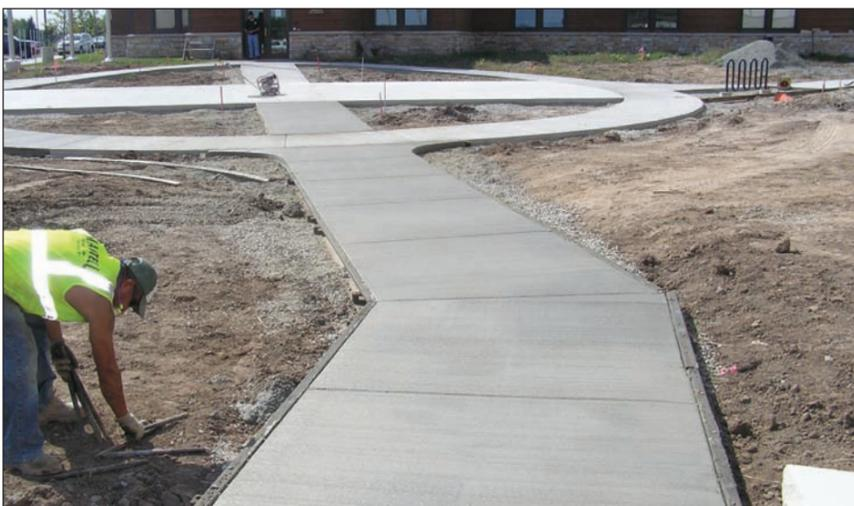
Josh Bailey removing pins and sidewalk forms for Martell Construction.
