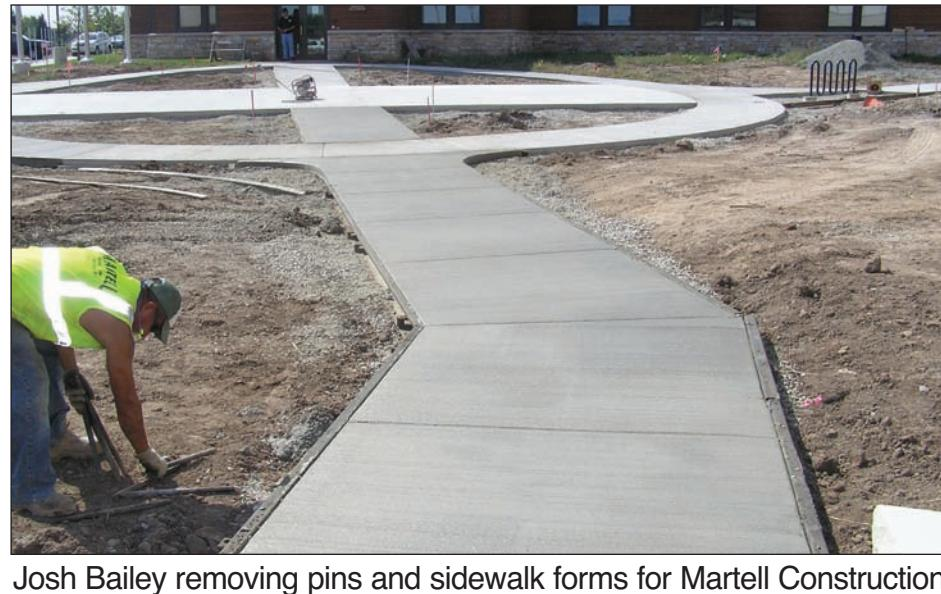
Josh Bailey removing pins and sidewalk forms for Martell Construction.
