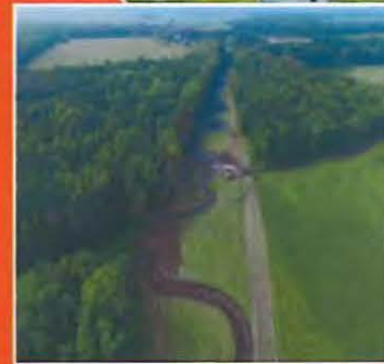
Tracking the progress of the S. Branch of the Suamico River restoration project.
