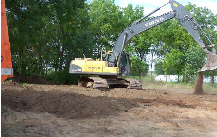
August 26, 2015 -DPW Staff finishing up demolation at the County C.
